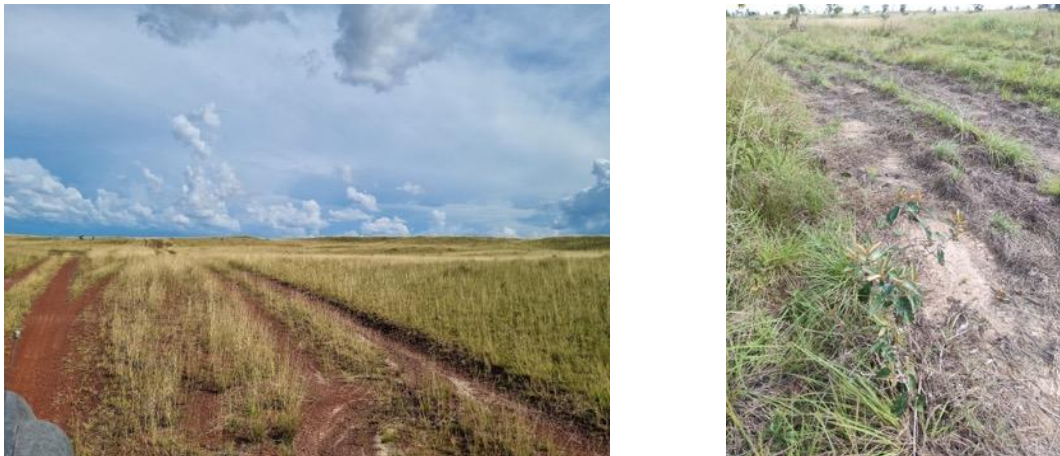
Figure 9 – Condition of the roads in the region.
